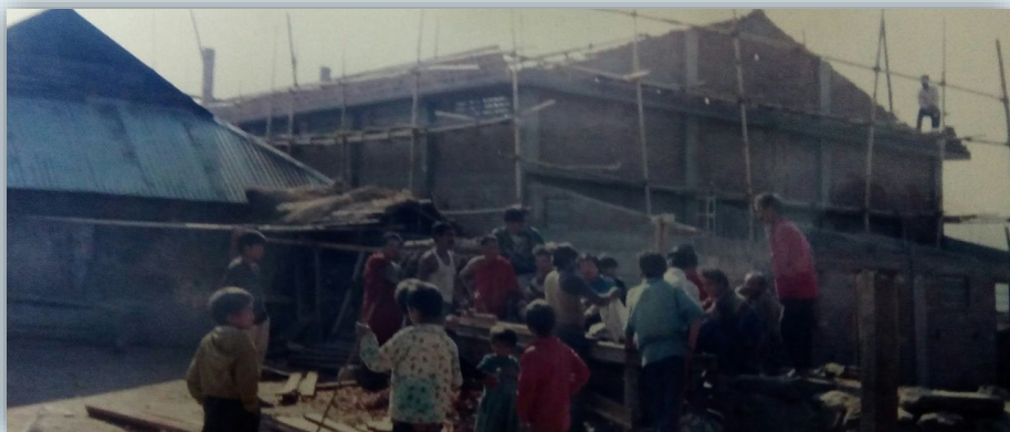
Church construction under progress, Kezoma.
